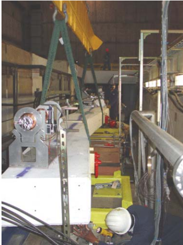
Figure 2: Installing the girder supporting the BPM3-5 triplet.
